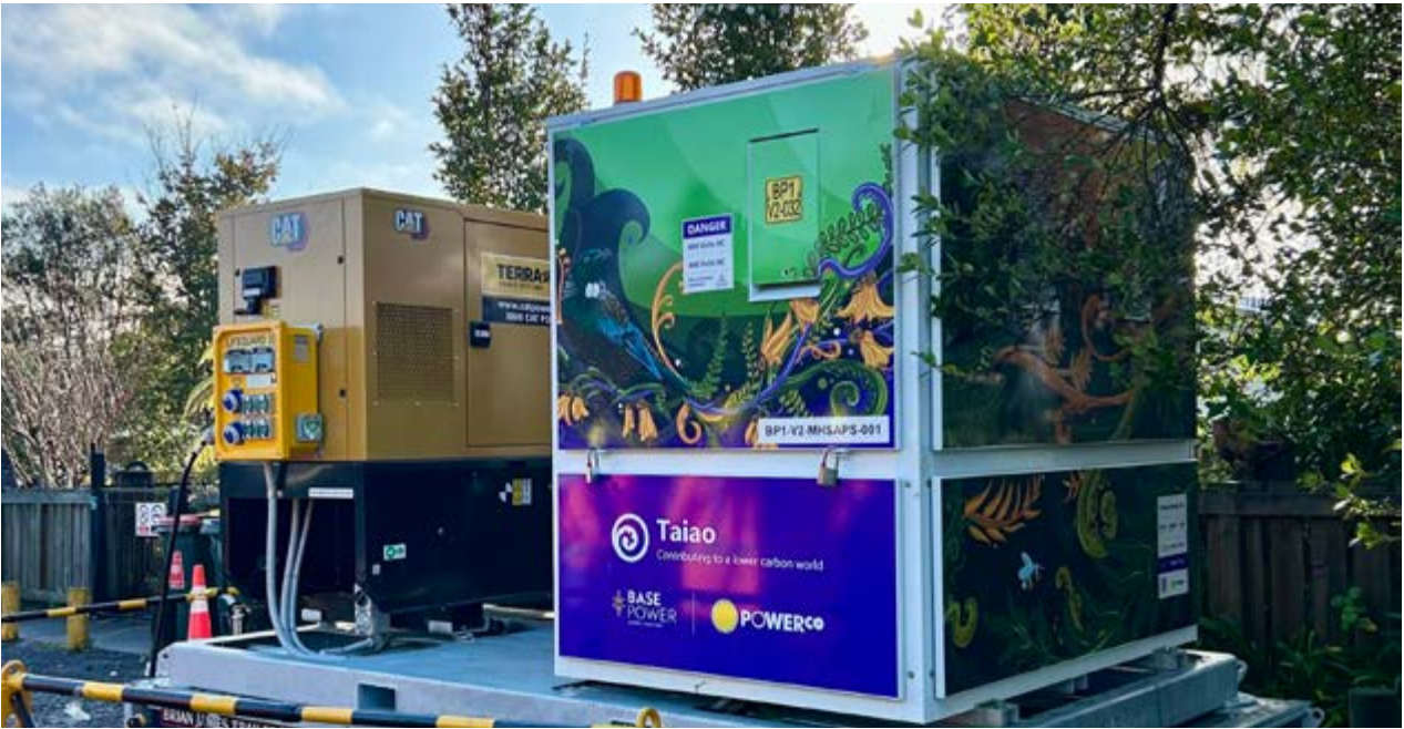
Powerco's mobile hybrid SAPS unit providing battery energy to a playcentre during a planned outage.
