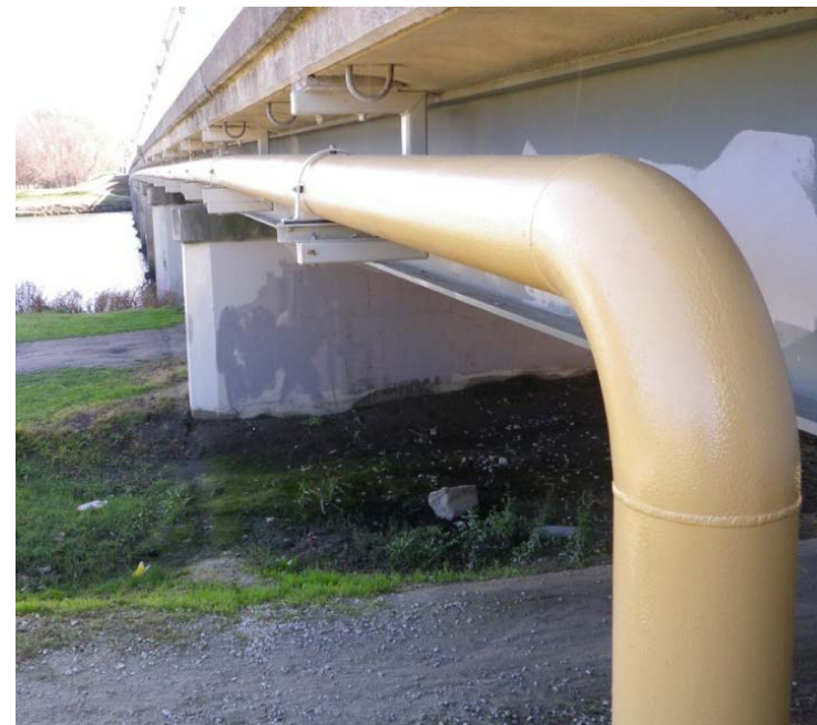
Figure 6.9: Bridge crossing in Hawke's Bay
