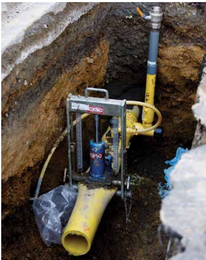
Figure 6.3: Pipe Repair Operation with Squeeze-off Equipment.
