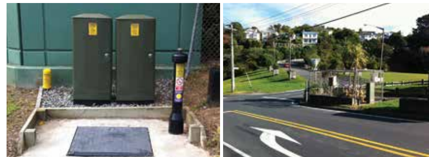
Figure 8.1: View of a Cocon Unit and an Above Ground Station.
