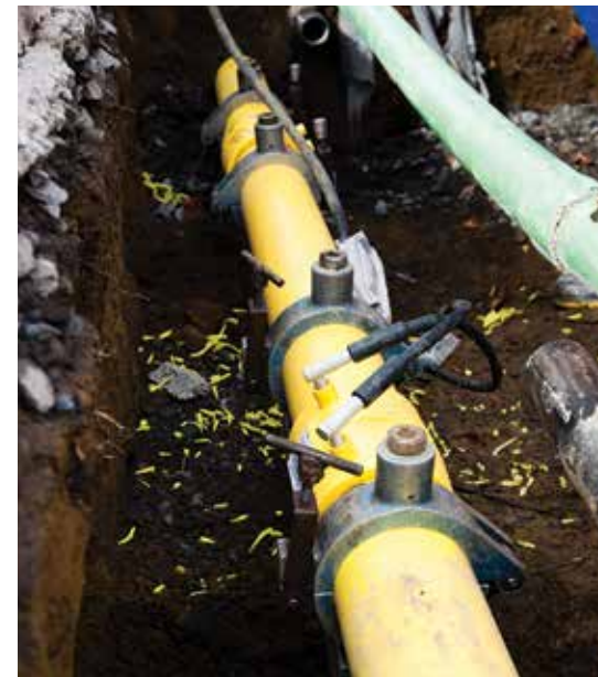
Figure 5.6: Electrofusion Operation to Joint Two Pipes.
