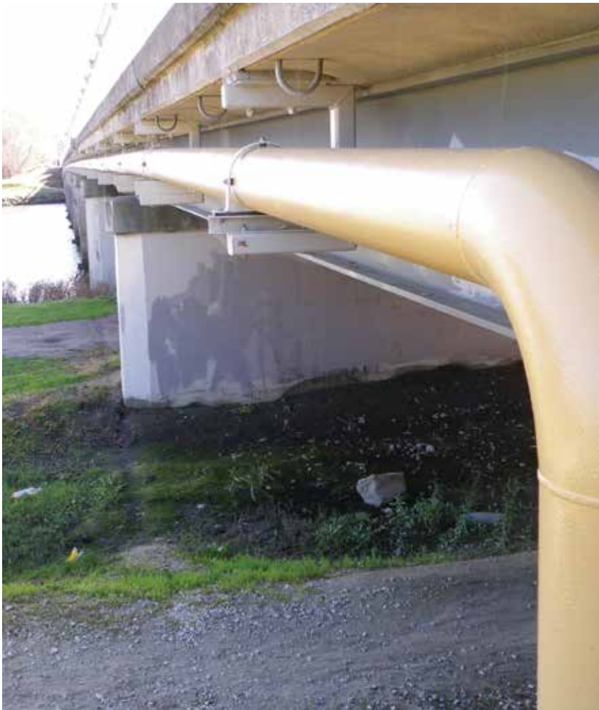
Figure 7.2: Bridge Crossing in Hawkes Bay
