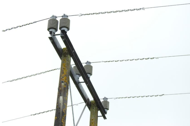
Figure 6 Enabling targeted use of Spiral Vibration Dampers designed to reduce the effects of aeolian vibration
