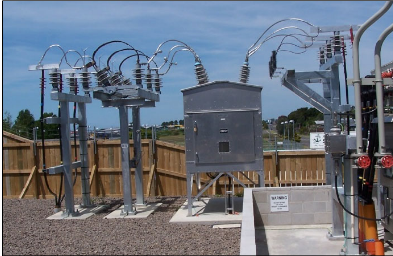
Figure 17.8: Typical outdoor 33kV switchgear bay
