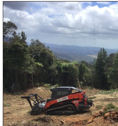
Eco-mulching provides a cost-effective way of creating a corridor around our subtransmission lines.
