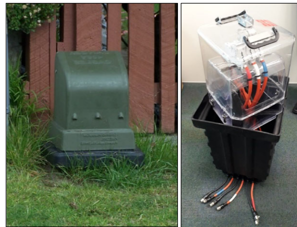
Figure 7.17: Example of organic adaptation. Standard LV pillars (left) are vulnerable to coastal inundation as they are not waterproof. A newer submersible design (shown right).
