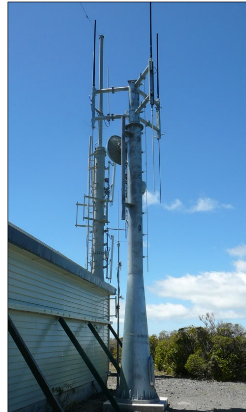
Figure 20.3: Communications mast with associated radio antennae
