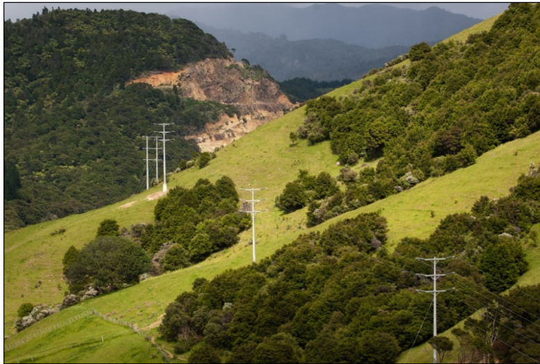
Figure 155.1: 66kV subtransmission overhead line in the Coromandel
