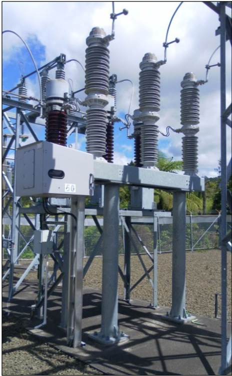
Figure 17.112: Live tank SF 6 outdoor 33kV circuit breaker
