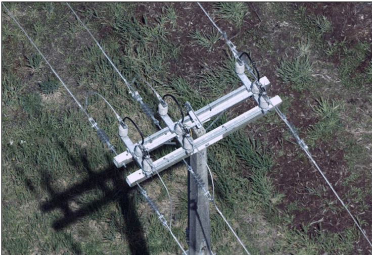
Figure 19.9: Air break switch (ABS)
