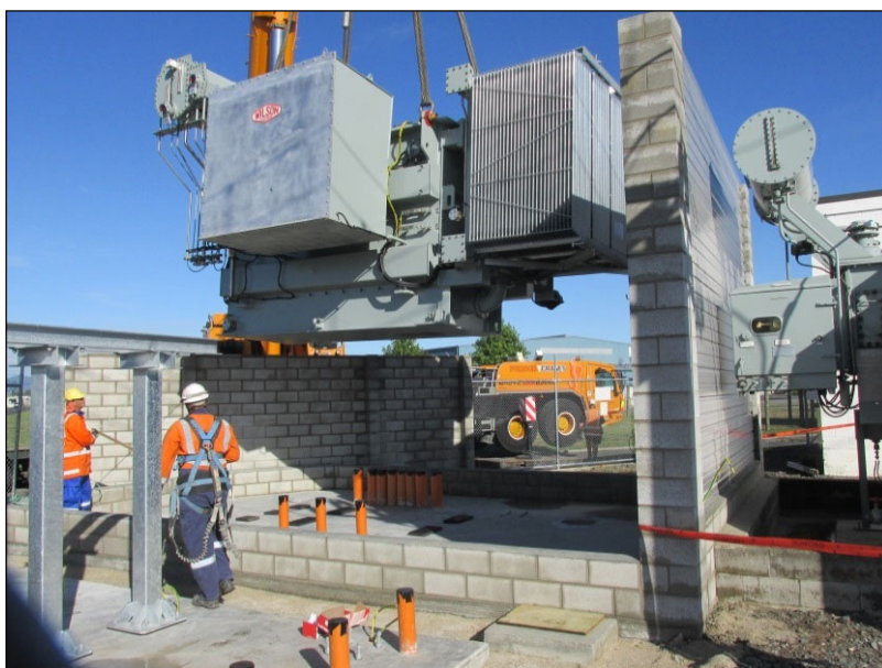
Figure 17.1: Power transformer installation at Waharoa
