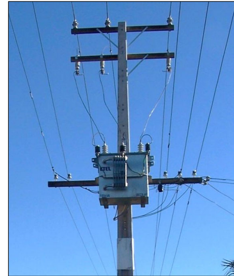
Figure 18.1: 100kVA pole-mounted transformer
