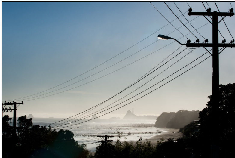
Figure 155.4: Distribution overhead line with LV underbuilt
