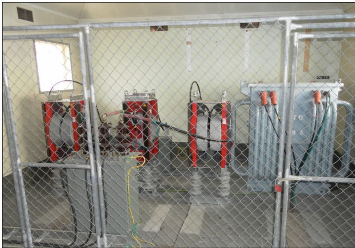
Figure 17.135: Load control injection plant
