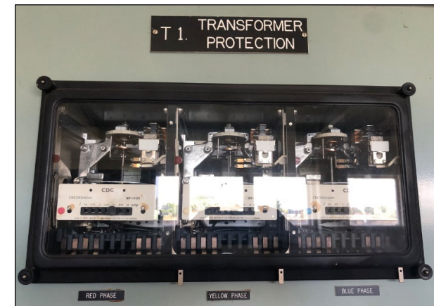
Figure 20.4: Electromechanical relays providing transformer protection
