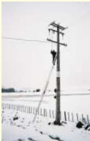
A Powerco Energy Services line mechanic restoring supply following a winter storm
