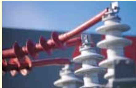
High-voltage transformer terminations
